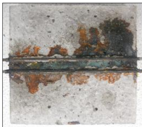
Figure 9. Photo of upper concrete surface and wires
